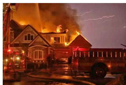
Lightning caused a home to become engulfed in flames in St. George, Utah, on Aug. 3, 2017. Photo by Nakavius Jaks, St. George News
